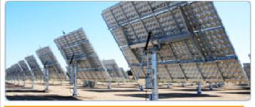
The first advantage of concentrator photovoltaic, due to multi-junction cells, is its efficiency. More than 40% for the cells in laboratory leads to a 25% panel efficiency, which is the highest energy yield of photovoltaic systems available today.
